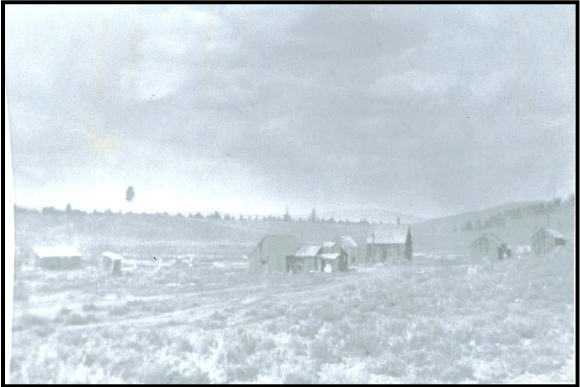
5. Unknown date, Old Joerger Ranch in Martis Valley, CA, when it was still operational. Facing northwest, structures from left to right: chicken house, privy, Mabel and Joe Joerger home, milk house, corrals, May and Roy Joerger home, boy's cabin (Lindström 2016, p.108).
